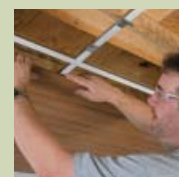
Position planks; slide and secure clips
